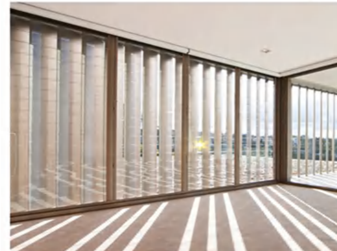
0-105° adjust the blade to control sun light
